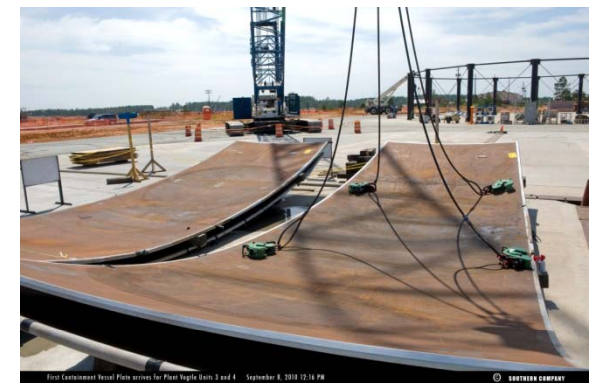
Containment vessel plate on site, Sept 2010
