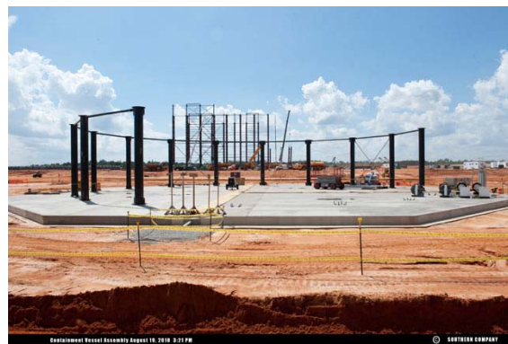
Containment Vessel Assembly, Aug 2010
